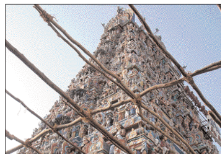
Kapaleeshwarar Temple's deity-clad roof
